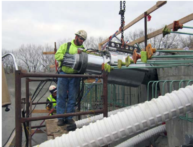
Figure 1.25 – Stressing Post-Tensioning Tendons
