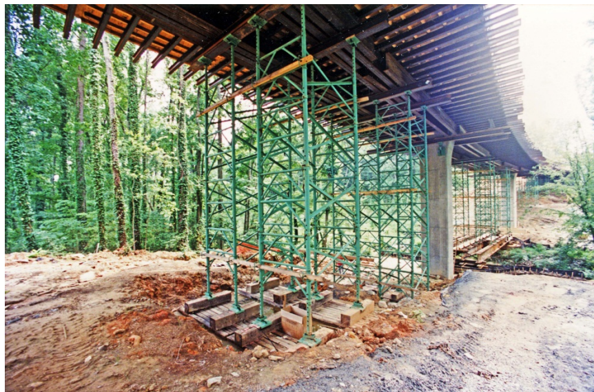
Figure 1.17 – Modular Falsework Units for Cast-in-Place Construction
