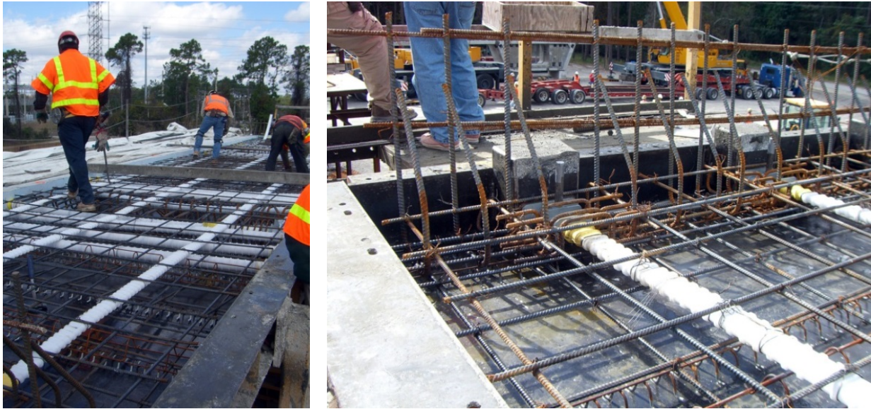
Figure 8.37 – Transverse Duct Placement in Casting Machine
