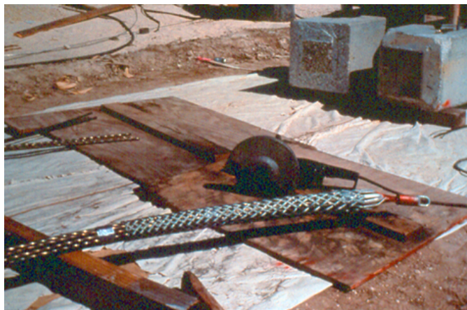
Figure 1.24 – Bundled Tendon Prepared for Pulling
