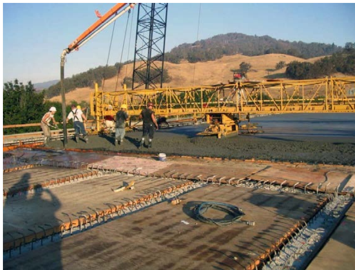
Figure 1.22 – Placing Deck Concrete and Finishing with a Roller Screed
