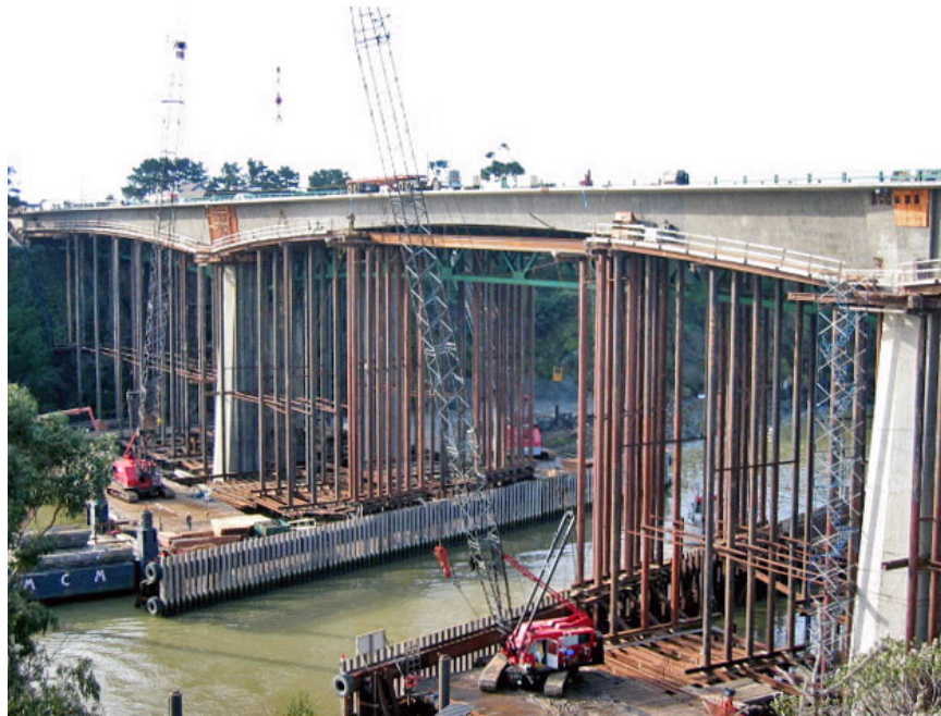
Figure 1.18 – Steel Pipe Support Towers for Cast-In-Place Construction
