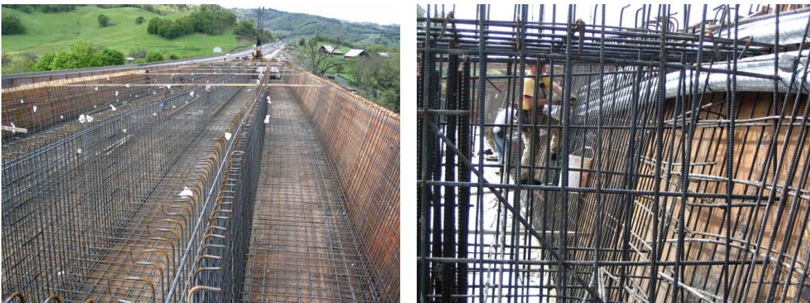
Figure 1.21 – Web and Bottom Slab Reinforcing (left), Tying Post-tensioning Ducts in Webs (right)
