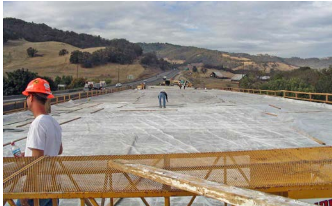
Figure 1.23 – Curing the Concrete Deck
