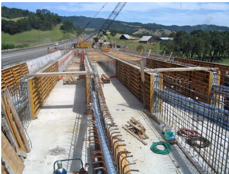
Figure 1.20 – Web Formwork for a Multi-Cell Box Girder
