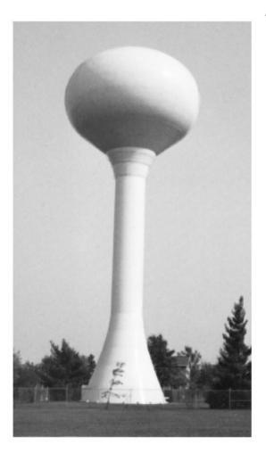
The column of the water tank shown in the figure is 300 ft high and is made of reinforced concrete with a tubular cross section of inner diameter 8 ft and outer diameter 10 ft. The tank weighs 6 x 10<sup>5</sup> lb when filled with water. By neglecting the mass of the column and assuming the Young s modulus of reinforced concrete as 4 x 10<sup>6</sup> psi, determine the following:
