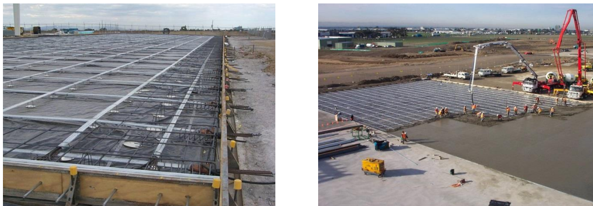
Figura 1.64 – Piso de concreto pós-tensionado. (Fonte: VSL, http://en.vsl.cz/joint-free-post-tensioned-slabs-on-grade )
