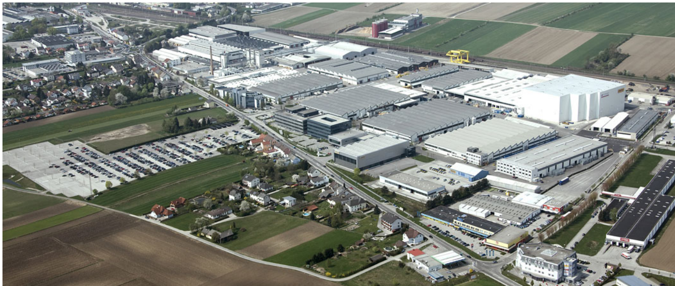
The Doka Group's central plant at Amstetten, Austria
