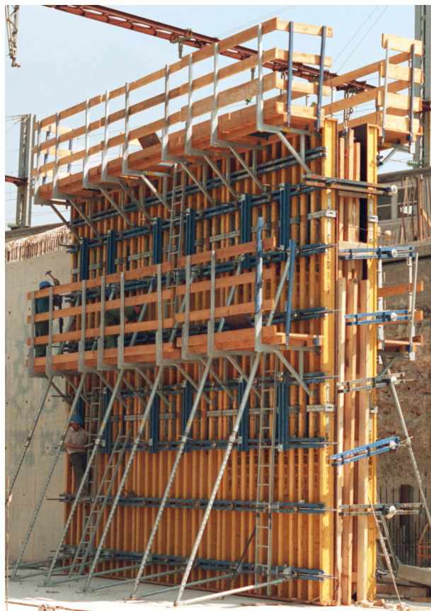
Obra: TVG Nord Bridge No. 4, Paris
