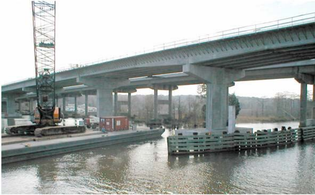
Figure 18. Photo. Precast spliced girder bridge.
