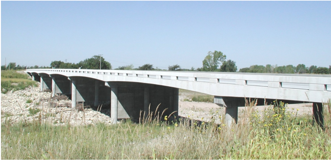
Figure 11. Photo. CIP PT concrete slab bridge.
