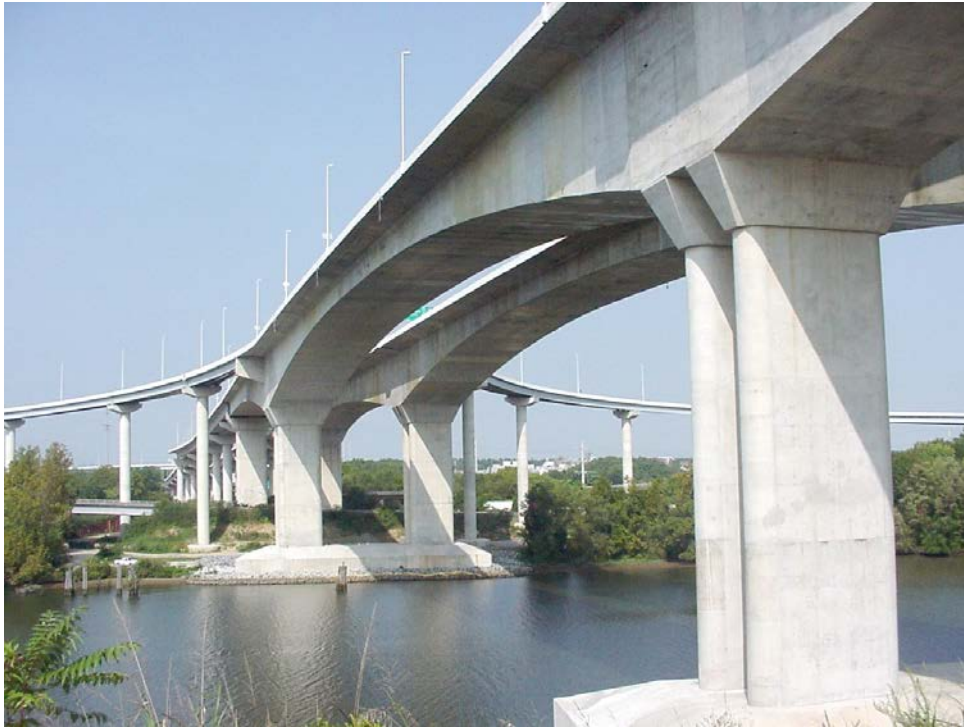
Figure 13. Photo. CIP segmental balanced cantilever bridge.
