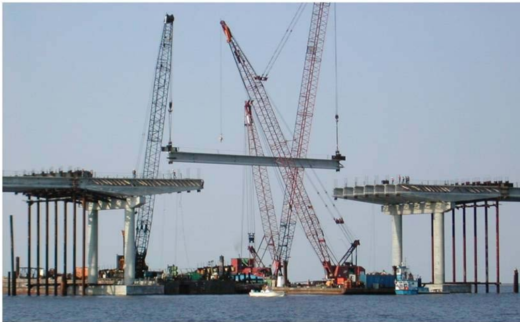
Figure 19. Photo. Precast spliced girder bridge during erection.
