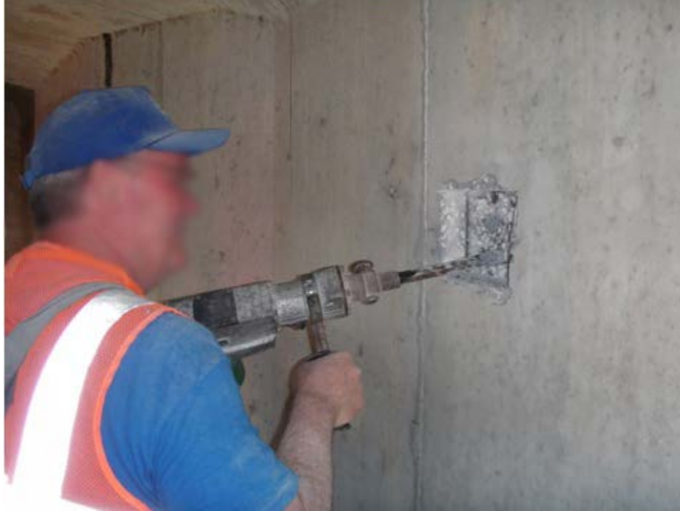
Figure 55. Photo. Concrete excavation to expose an internal tendon.
