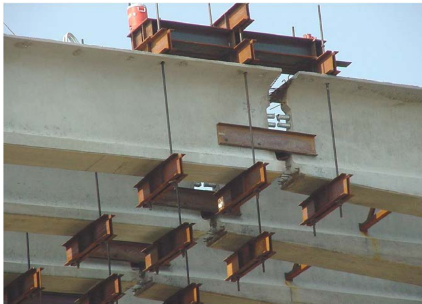
Figure 70. Illustration. Spliced bulb-tee girder bridge inspection point locations.
