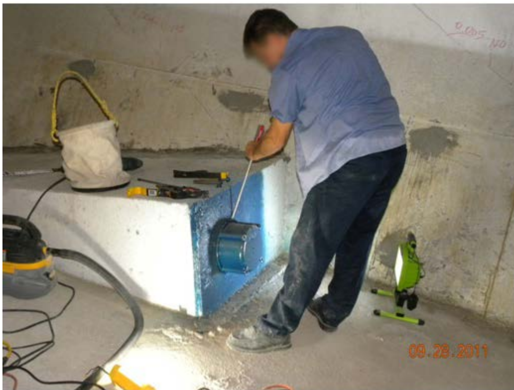
Figure 62. Photo. Removing a permanent grout cap.
