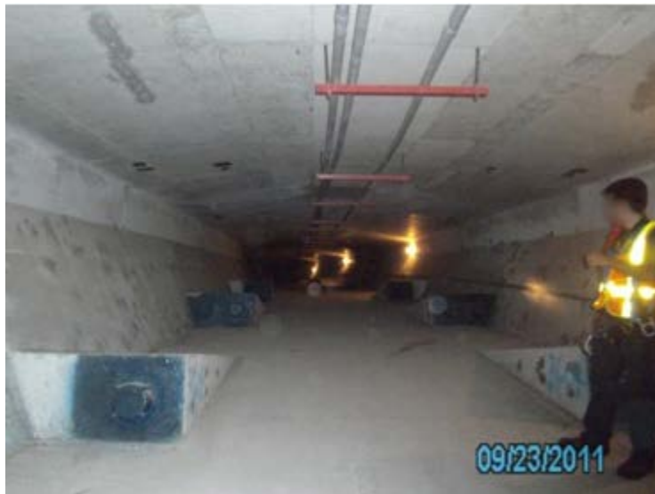
Figure 15. Photo. Typical bottom flange blister.
