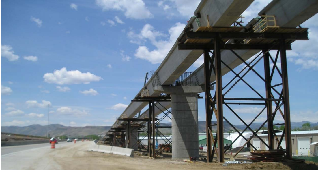
Figure 21. Photo. Precast U-girder supported on temporary false work.
