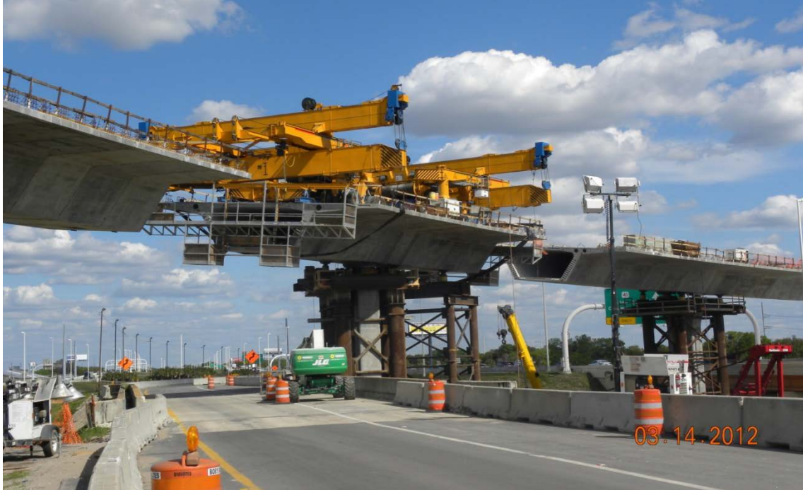
Figure 22. Photo. Precast segmental balanced cantilever bridge erection using a segment lifter.
