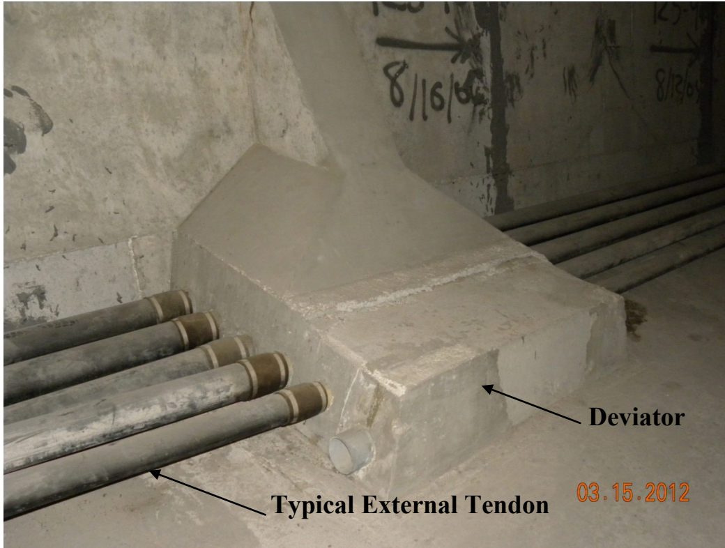
Figure 6. Photo. External tendons at deviator.
