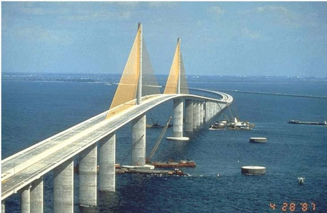
Figure 25. Photo. Precast segmental cable stayed bridge.
