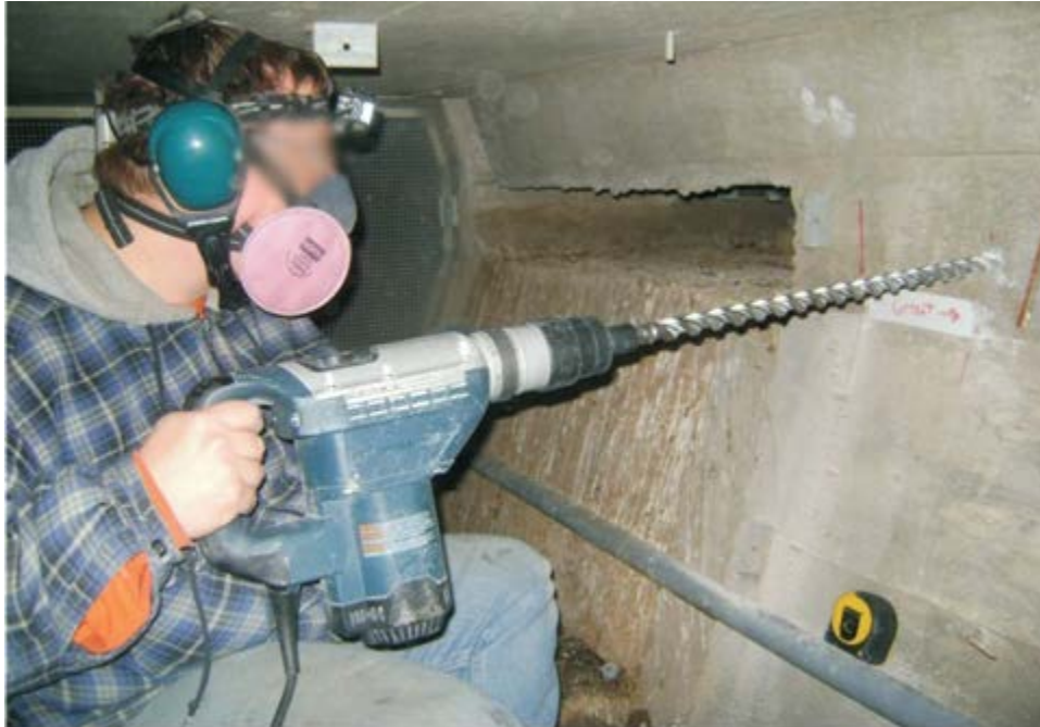
Figure 56. Photo. Internal tendon access at an intermediate location by drilling.
