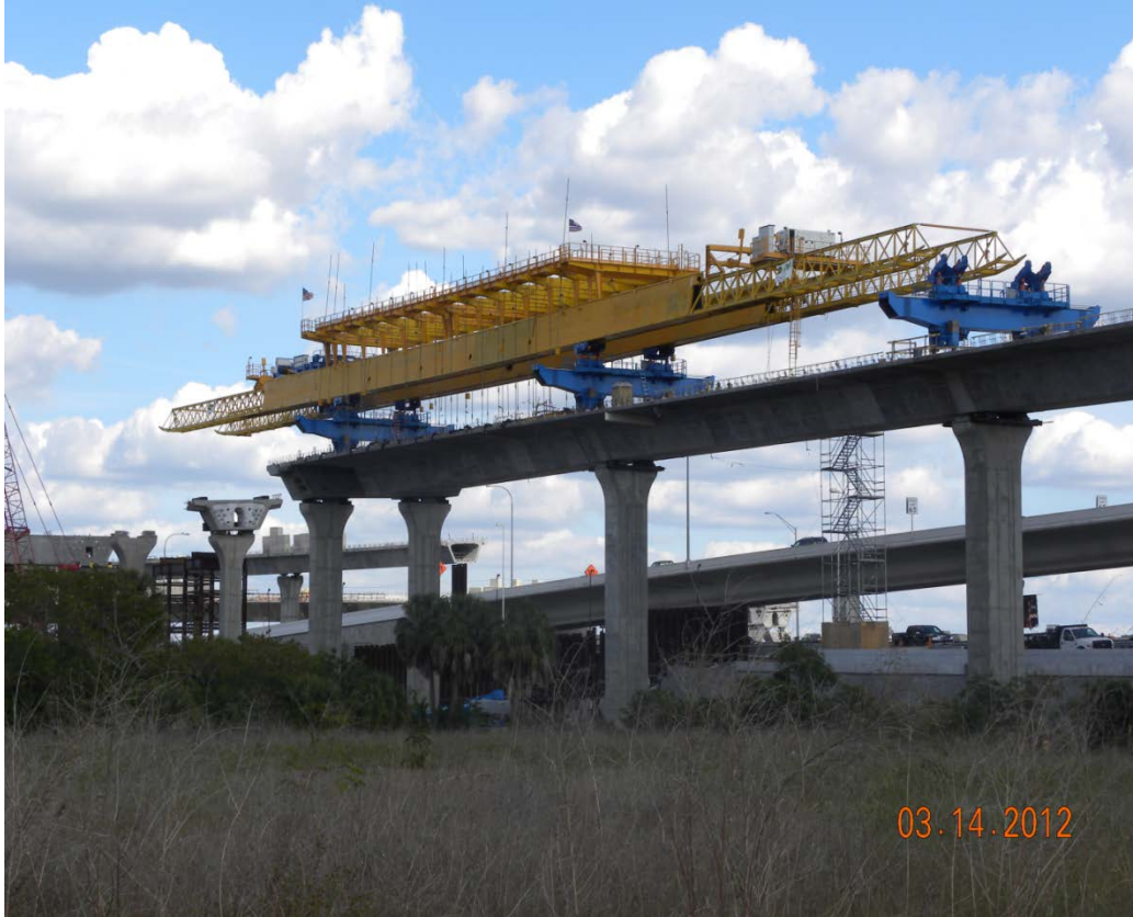
Figure 23. Photo. Precast segmental span-by-span erection using an overhead gantry.
