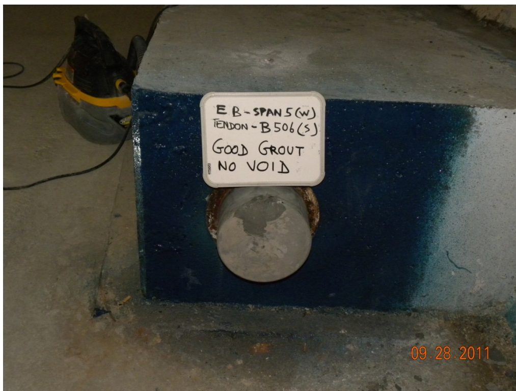
Figure 63. Photo. Exposed anchor head after grout sampling.
