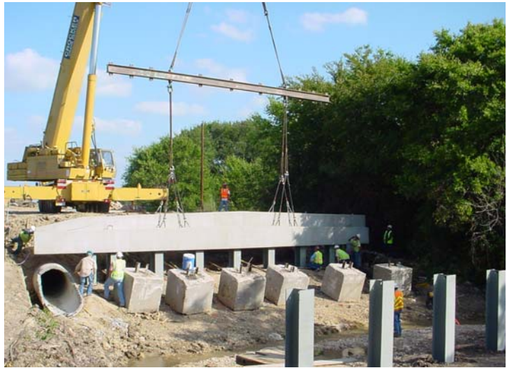
Figure CS3-4 Abutment Bent Installation
