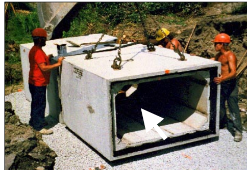
Image Courtesy American Concrete Industries, 2007
