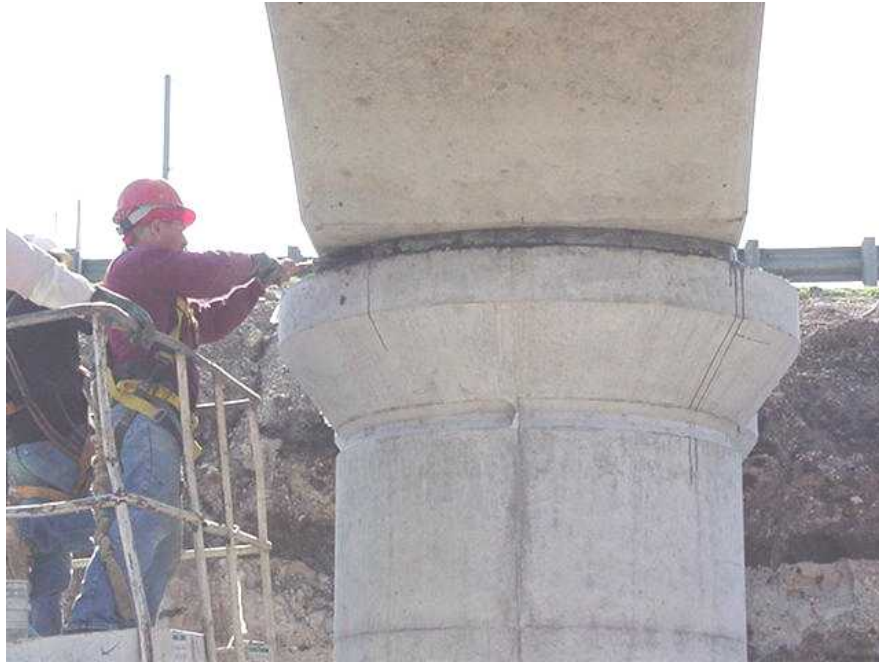
Figure CS2-7 Dry Pack Grouted Placement
