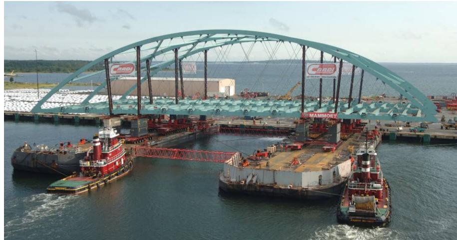
Figure 1.8.3.2-1 Providence River Bridge (Photo Courtesy of Mammoet)
