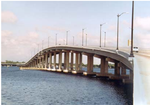
Figure EX3-2 Edison Bridge
