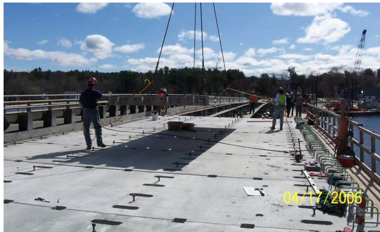
Figure 1.2.4-1 Full Depth Precast Deck Panels
