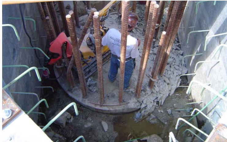
Figure 4.1.7-2 Providence River Bridge Pier Box Preparation for Footing Reinforcing Placement
