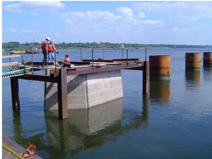
Figure 4.1.7-1 Providence River Bridge Pier Box
