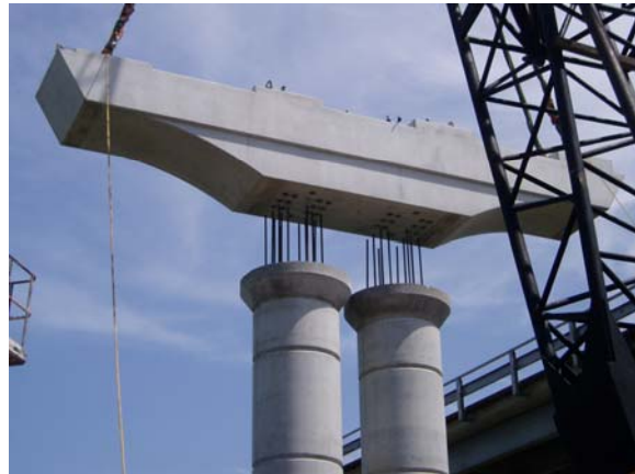
Figure EX2-1 Lake Belton Bridge Pier
