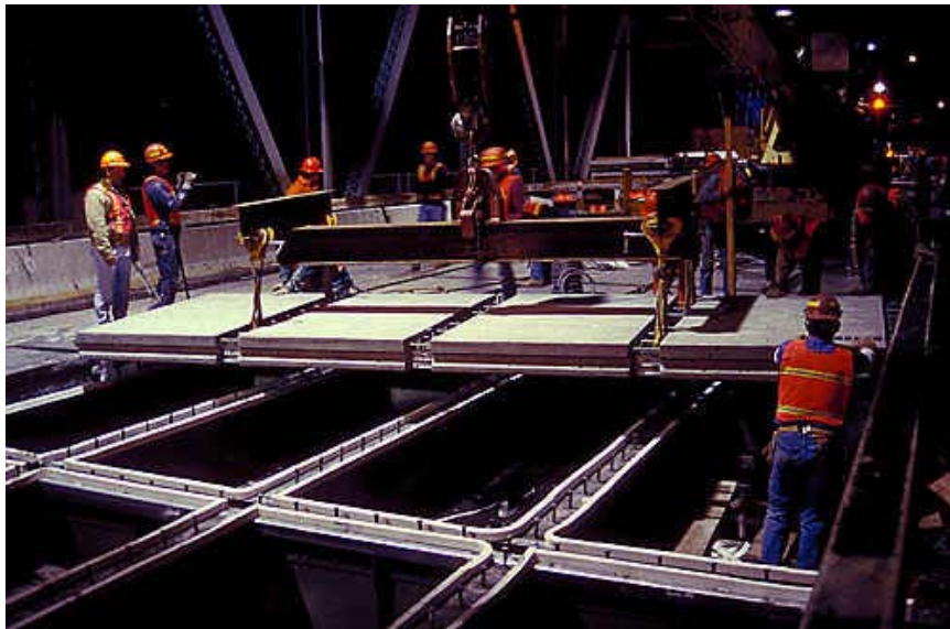
Figure 2.1.3-2 Exodermic Deck Installation Photo courtesy of the D.S. Brown Company
