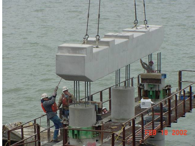
Figure 1.2.4.-2 Precast Pier Cap
