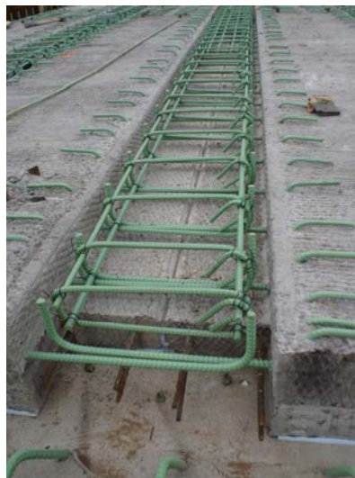
Figure 2.2.3.1-1 Minnesota Adjacent Beam System
