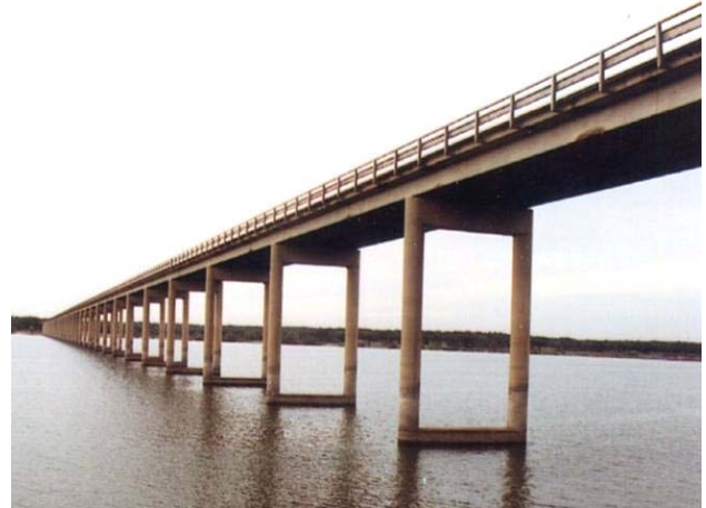
Figure CS2-1 Existing Bridge
