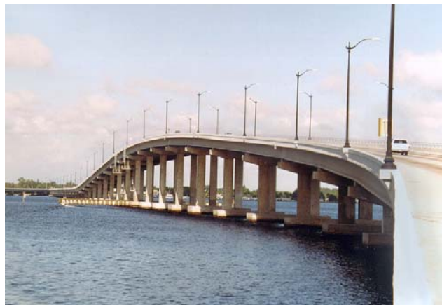
Figure CS4-9: Edison Bridge
