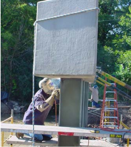
Figure CS3-3 Pile to Cap Connection
