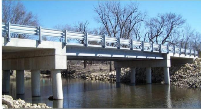
Figure 15. Photo. Jakway Park Bridge, Buchanan County, IA
