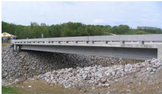
Figure 13. Photo. Mars Hill Bridge, Wapello County, IA
