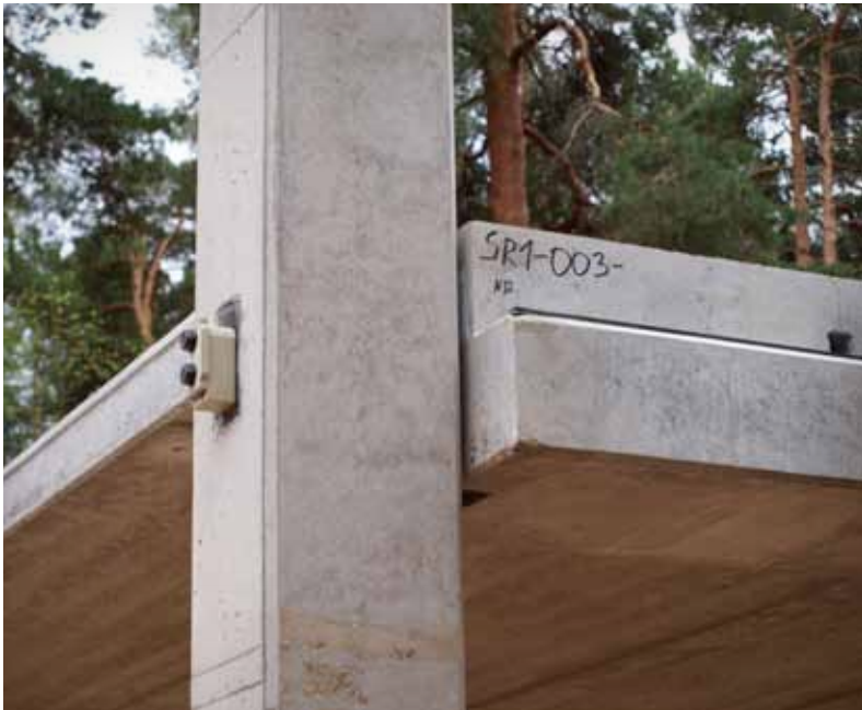
Precast Column and Inverted Tee Connection with Hollowcore— Isometric view
