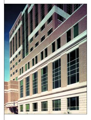
• Smaller stone inserts can be cast as "highlights" in larger precast panels.
