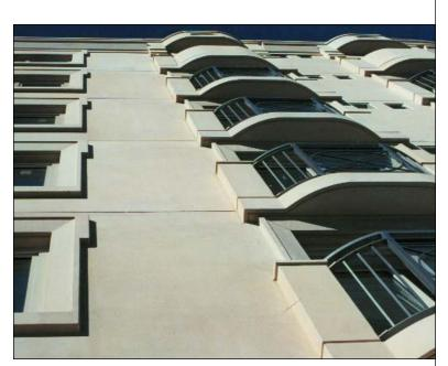
solution; by spraying an acid and water mixture onto the panel surface; or by immersing the precast unit itself into a tank containing a solution of hydrochloric acid. Subsequent thorough washing of the panel to flush the acid residue from the panel surface must be done to prevent a continued reaction of acid with panel components.
