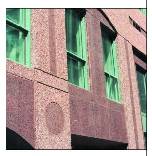
sections are more economically assembled as veneer units on precast concrete panels.
