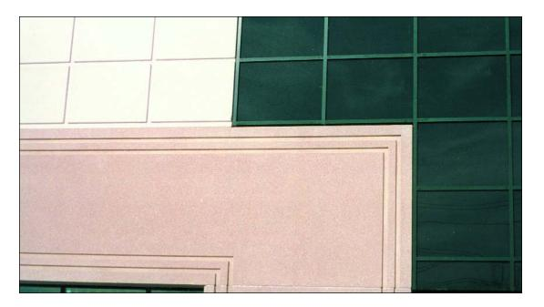
be controlled within the limits of strength and absorption requirements and not exceed 6% by weight of cement. Different shades of colour can be obtained by varying the amount of pigment or by combining two or more pigments. White Portland cement will produce cleaner, brighter colours and should be used in preference to grey cement, especially for the light pastels such as the buffs, creams, and ivories, as well as the bright pale pink and rose tones.
