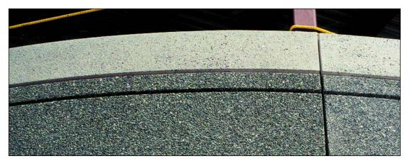
show any obvious imperfections other than minimal colour and texture variations, nor should it provide evidence of repairs when viewed in typical lighting with the unaided naked eye at a 6 meter viewing distance. Appearance of the surface should not be evaluated when sunlight is illuminating the surface from an extreme angle, as this tends to accentuate minor surface irregularities.
